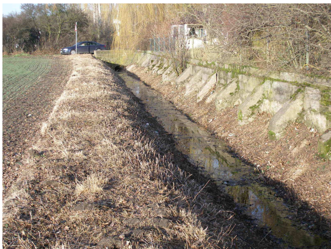
Abb. 1: Bestandssituation an Station 26,50 m
