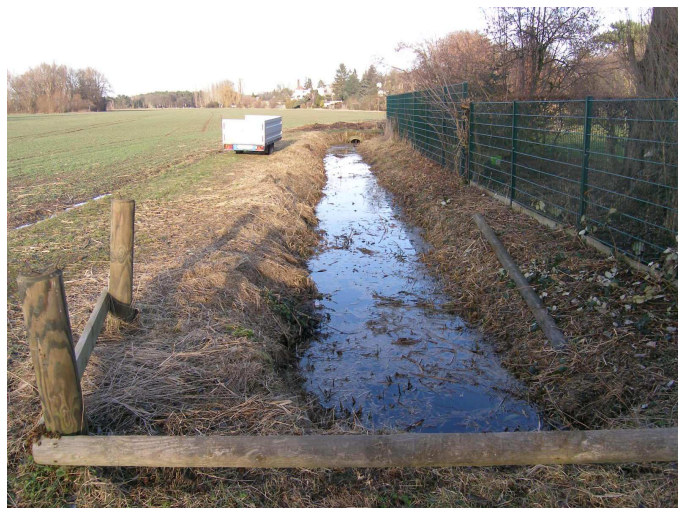
Abb. 2: Bestandssituation an Station 468,00 m
